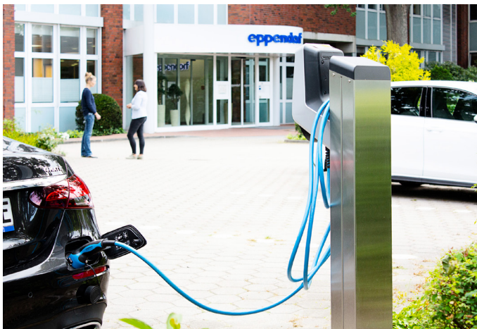
Figure 4: Car charging stations at Eppendorf headquarters, Hamburg, Germany
